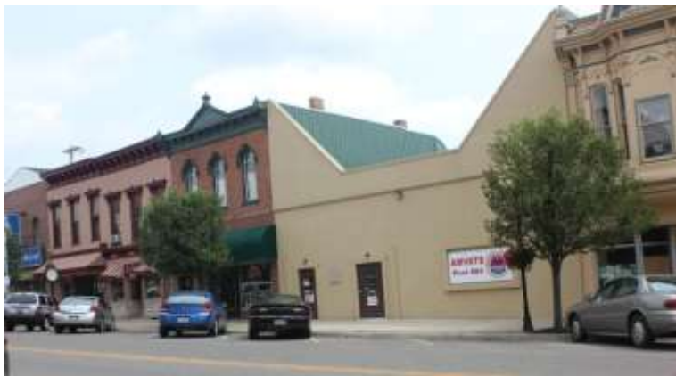
Figure 14: This image illustrates an infill building that would not comply with these standards of new construction in terms of height, roof styles, window and door patterns, siding, ornamentation, signage, and most other requirements in the Restoration District.
