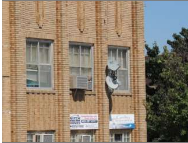
Figure 1: Satellite dishes, air-conditioning units, and similar equipment shall be located on the roof or to a side of the façade not visible from public rights-of-way, to the maximum extent feasible.
