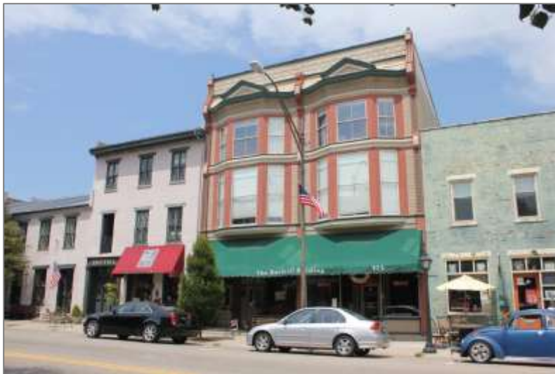
Figure 7: The Burwell Building contains a number of architectural ornamentations that should be maintained during any future work on the building.
